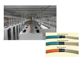
In case of a Fire, Most people dies due to the smoke and gases emanated by PVC jacketed cables. We encourage our customers to use our cable solutions that do not contain any halogen, therefore they do not emit toxic and corrosive fumes when burning and only a minimum amount of smoke
